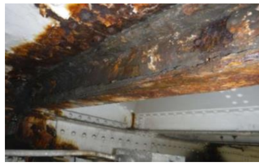
Vauxhall Bridge (steel fatigue / overall condition – very poor) Daily users – 47,000
